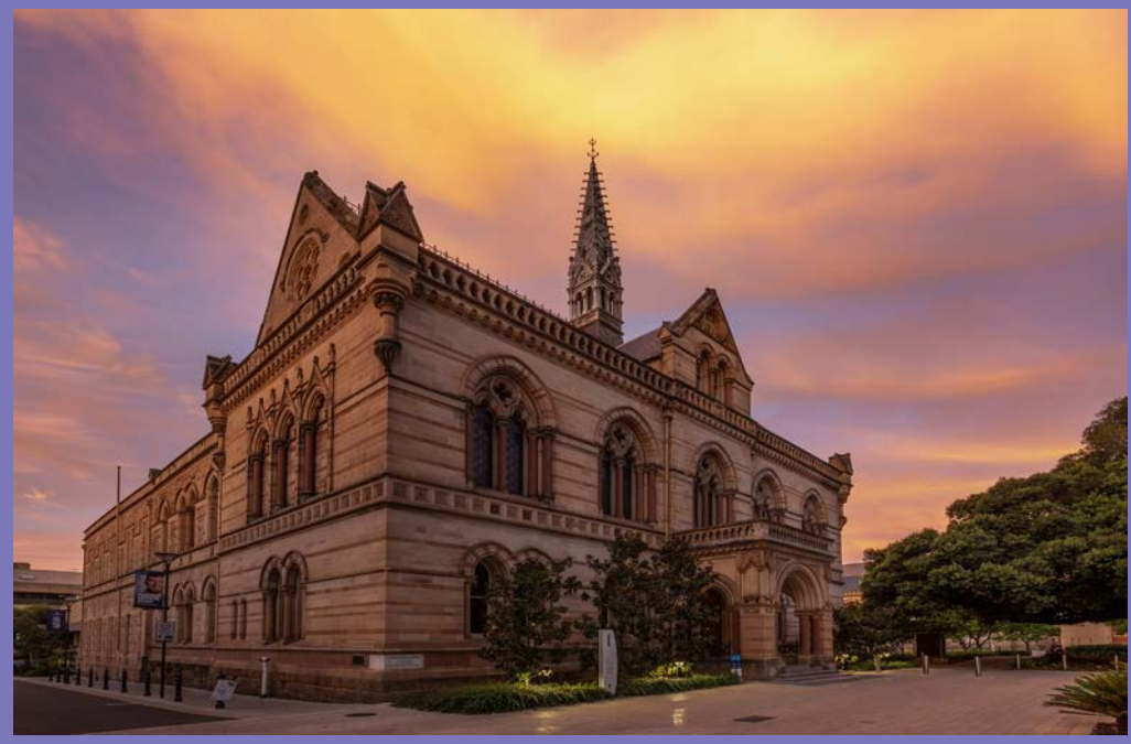
Michael Waterhouse Photography - North Terrace, Adelaide
